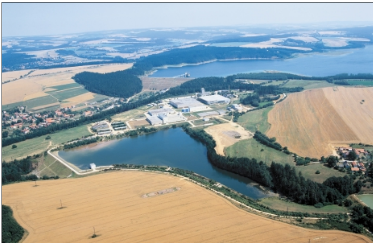
□ Želivka water storage reservoir operated by Pražské vodovody a kanalizace, a. s.
